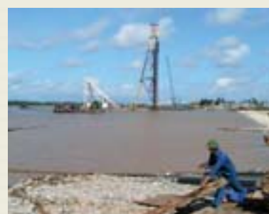
Construction work in progress at Hai Phong Port
