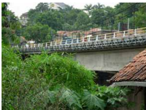
Sasakbeusi Bridge, West Java Province
