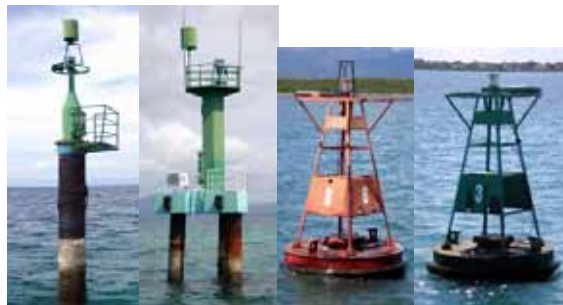
Beacons and lighted buoys
