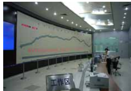
Traffic Control Center in the Liangping toll plaza of Wanxian-Liangping Expressway
