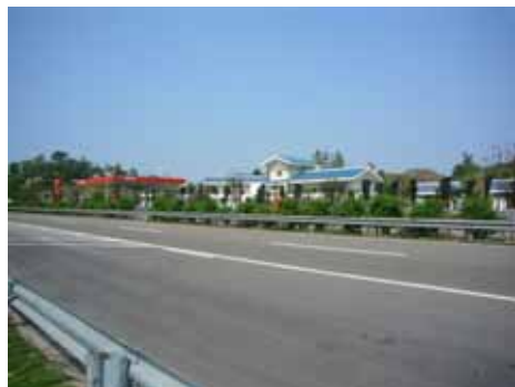
Liangping Service Area, Wanxian-Liangping Expressway
