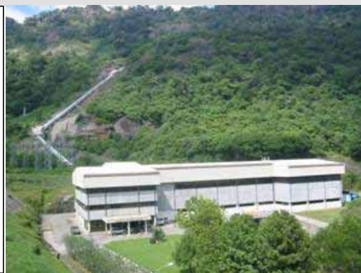
Samanalawewa Hydroelectric Power Station Control Building
