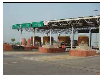
Toll booths on the Naini Bridge
