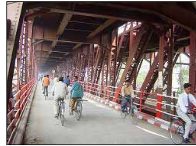
Yamuna Bridge (old bridge)
