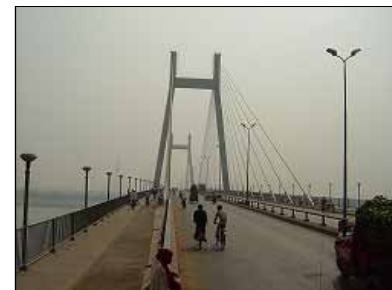
Naini Bridge (new bridge)
