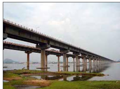
NH-5, Krishna Bridge (Phase I) Vijayawada, AP State
