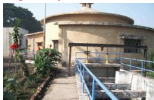
Sewerage Pumping Station
