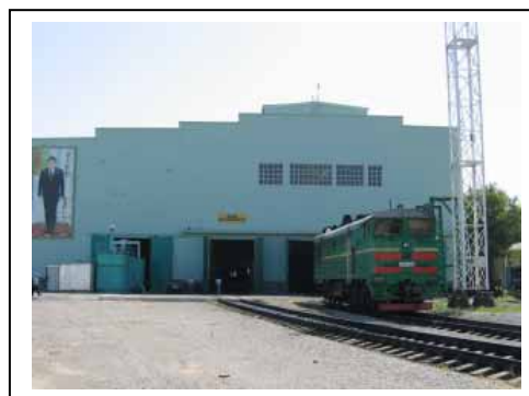
Exterior of Locomotive Repair Workshop
