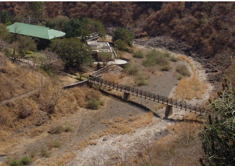
(Figure 18) Newly built bridge at the foot of the site
