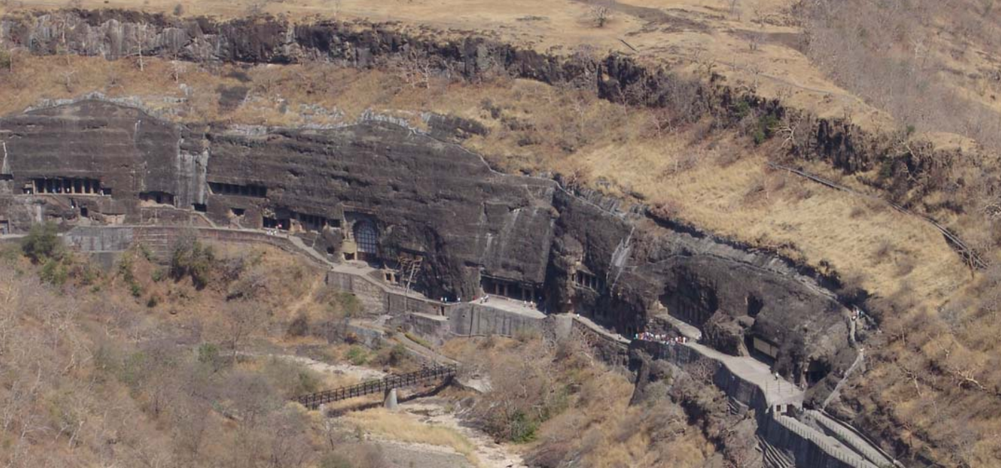
(Figure 20) Drainage maintenance work
