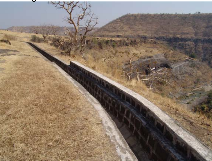
(Figure 21) Drainage system installed on a flat surface above the caves
