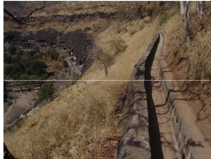
(Figure 22) Drainage system at the bottom of the cliff
