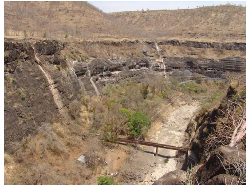
(Figure 19) Old bridge in the back of the historic site
