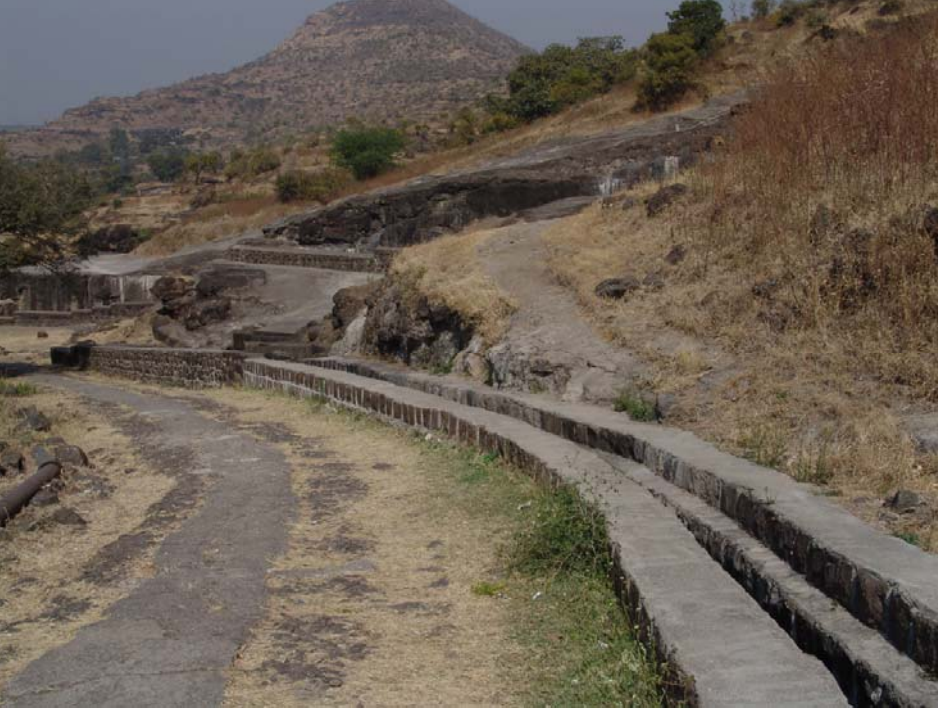
(Figure 49) Drainage maintenance work Above cave 16 (left), drainage system carrying water from above cave 1 to side of cave 16
