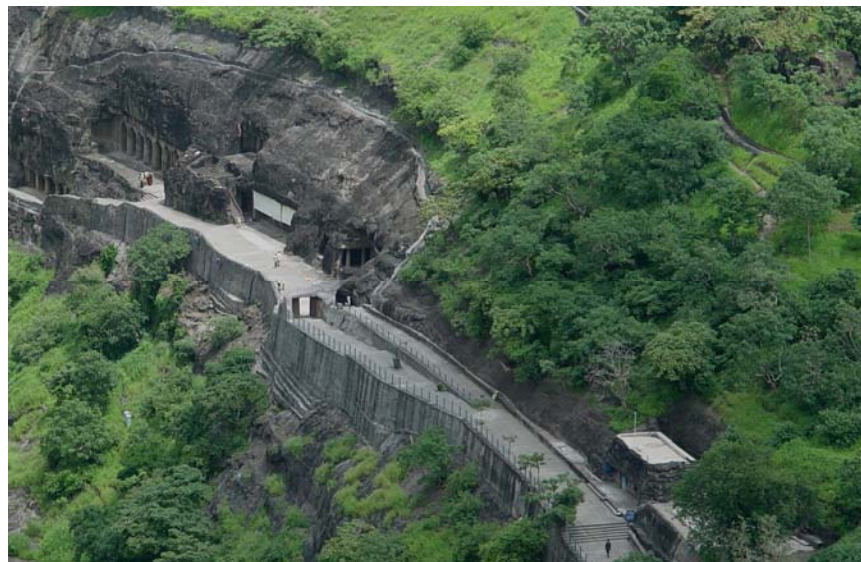
(Figure 11) Retaining wall that resembles a defensive wall
