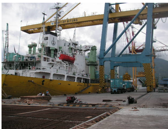
Loading at Completed Container Berth of Bitung Port
