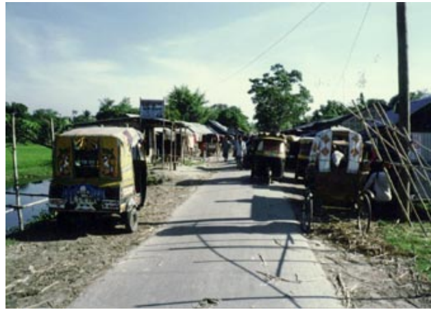
Road established by Model Rural Development Project. It has become a mini-cab depot
