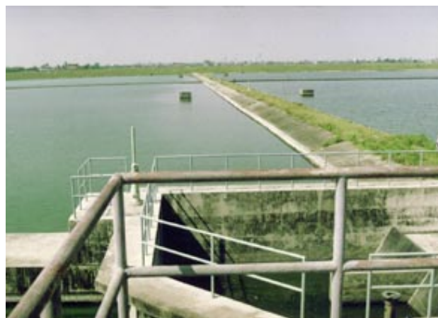
A lagoon constructed through construction and rehabilitation of the sewerage
