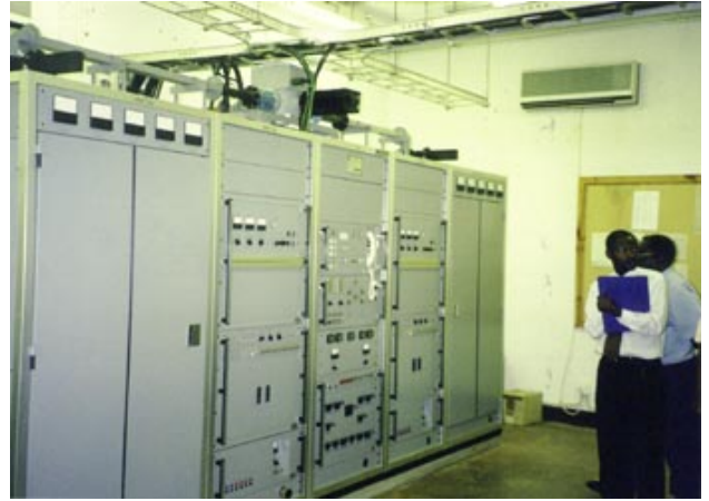
A repaired observation system
