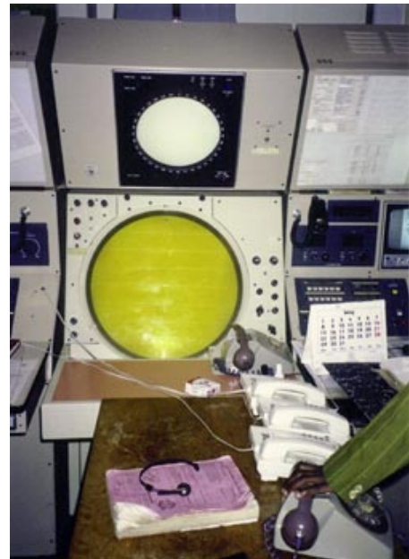
A newly replaced air control radar
