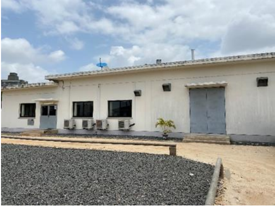
Control building (Ilala substation)
