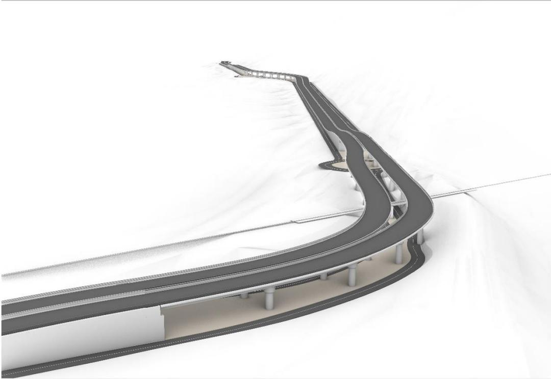
**Figure 4-7** 3D Representation of the First Flyover Section over Nakuru's 1<sup>st</sup> Roundabout with a view on the at Grade section
