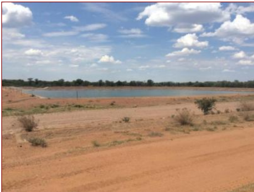
Figure 21- Northern dam associated with the AFD
