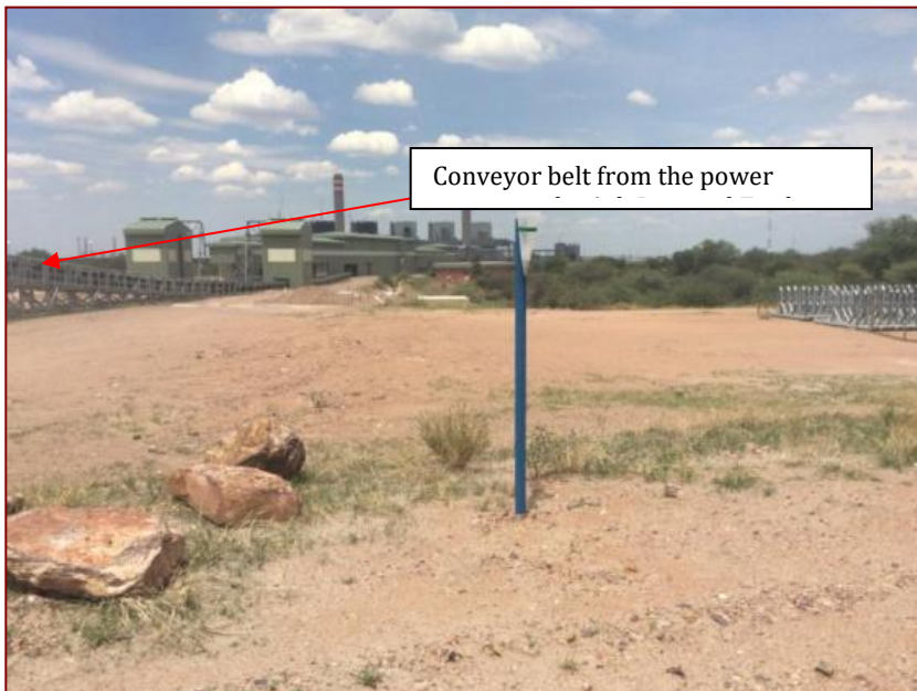
Figure 23- Conveyor belt system associated with the AFD
