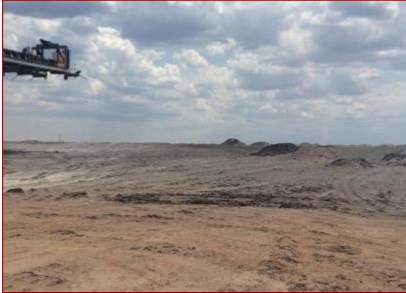
Figure 22- Current ash heap at the ADF facility
