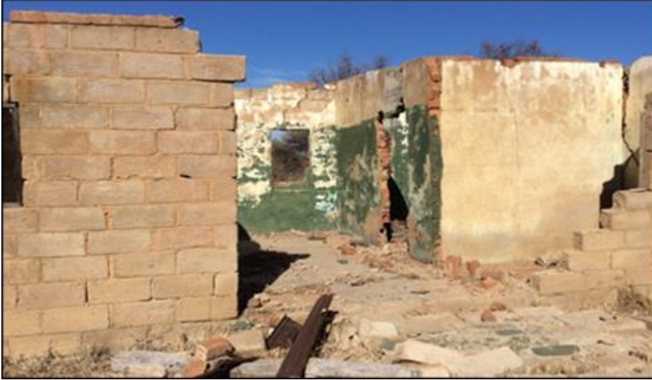
Figure 9-Remains of old brick structure on site 12.
