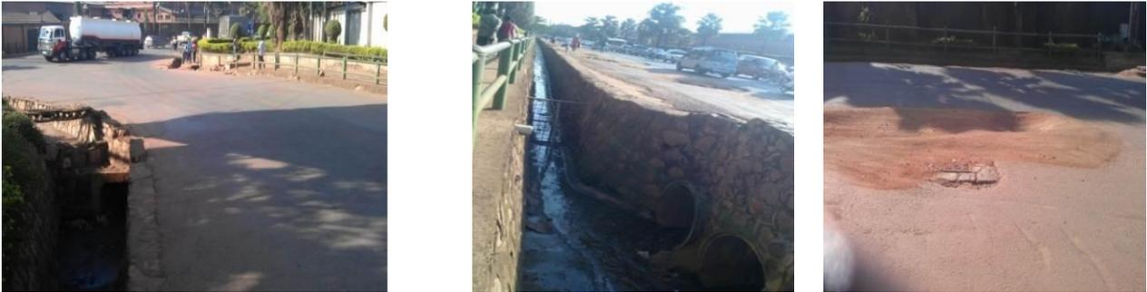
**Photo 5-7: The drainage of the area. The pothole shown is probably as a result of some water ponding on the road surface as opposed to running into the drain.**
