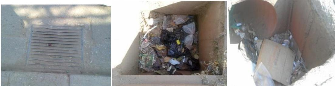
**Photo 5-3: Blocked Drains and Waterways around the Clock Tower Area (August 2013)**
