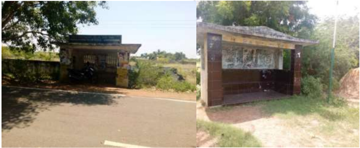
Figure 6-1 Photos pf Affected Bus Bays
