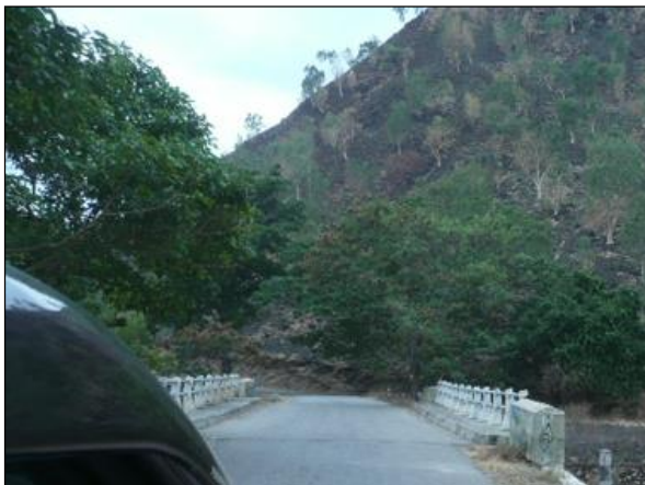
Photograph 3 Dili to Manatuto – Km 40.5 Lainlidum Bridge
