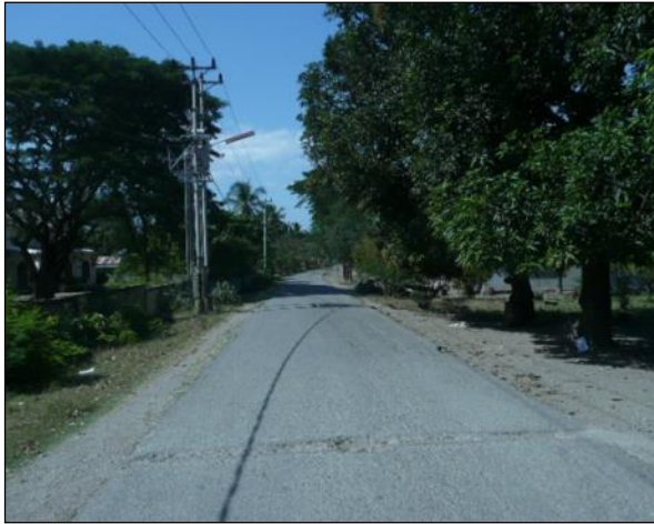
Photograph 1 Hera to Manatuto – Km 9.3 Police Station
