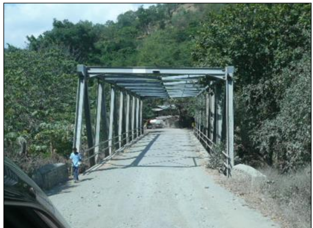
Photograph 5 Dili to Manatuto – Km 48.0 Beheda Bridge
