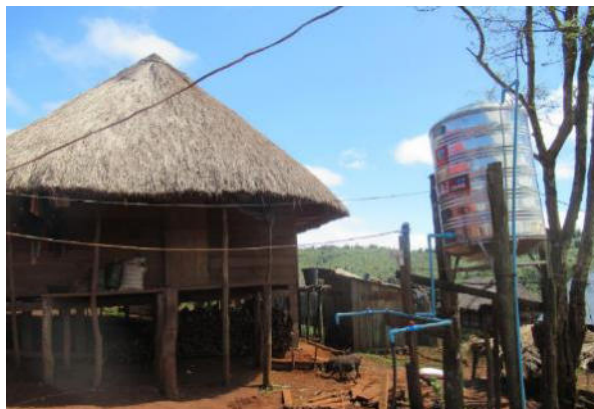
Water storage tank in Dak Yen Village
