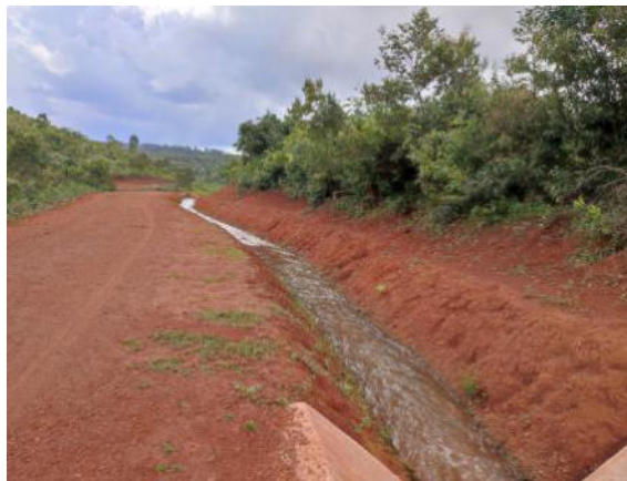
Irrigation in Dak Rant Village
