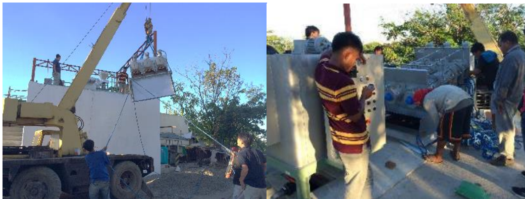
Photo: Scenes from the installation of the dewatering equipment
