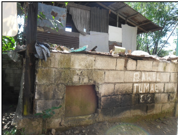
Structures to be additionally demolished at CP-III
