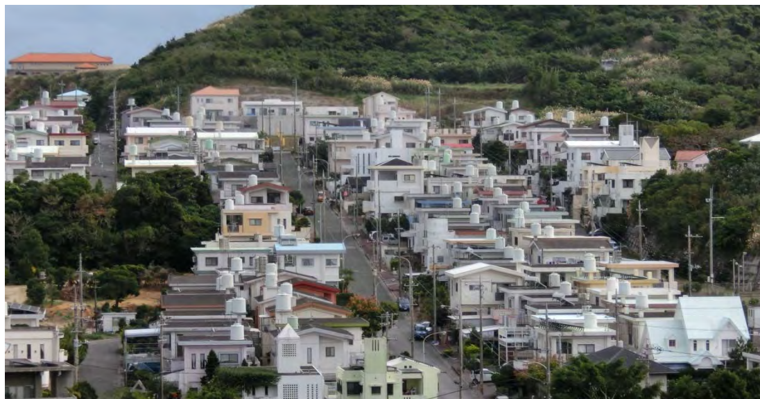
Photo 2. Rooftop Tanks in Okinawa Prefecture (December 28, 2016)
