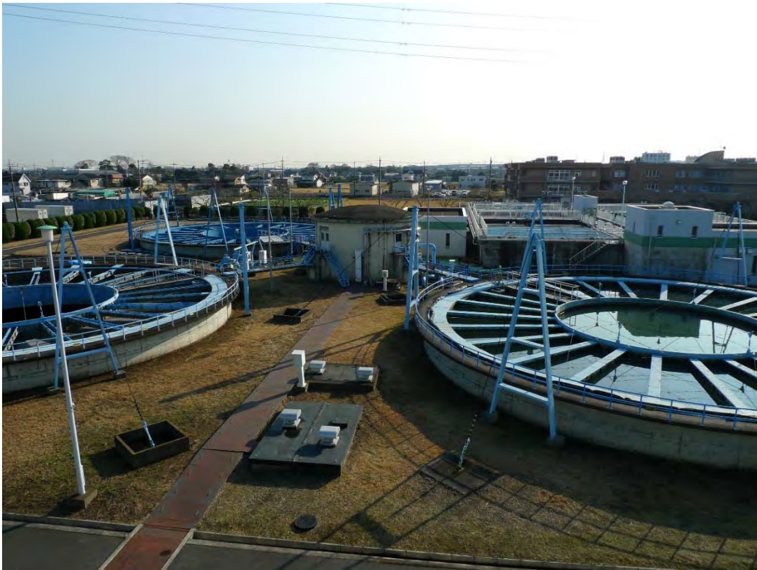
Photo 2. Kakinoki Water Treatment Plant (December 22, 2010)
