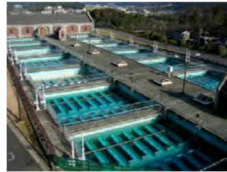
The first plant using rapid sand filtration in Japan (Keage WTP, Kyoto City)
