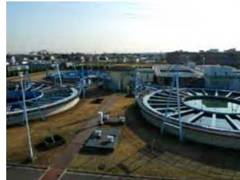
Kakinoki purification plant
