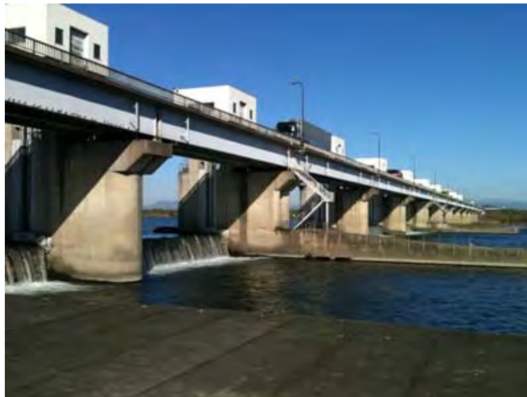
Photo 4. Tone Ozeki; Water intake facilities of the Musashi Channel (November 19, 2010).
