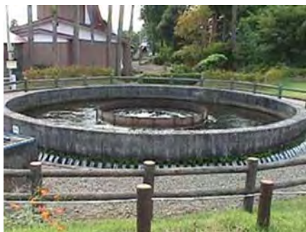
Cylindrical Siphon to allocate water equally, built in 1938 at Rokugou town, Akita Prefecture http://www.pref.akita.jp/fpd/tuchi/nanataki.htm
