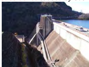
Multi purpose dam
