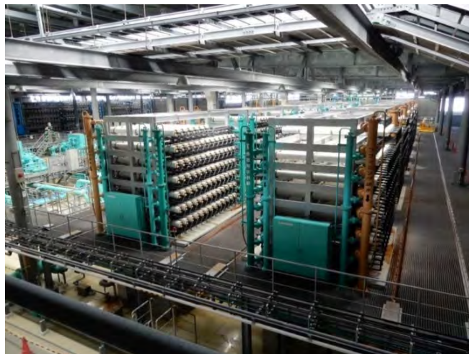
Photo 4. Uminonakamichi Nata Sea Water Desalination Center
