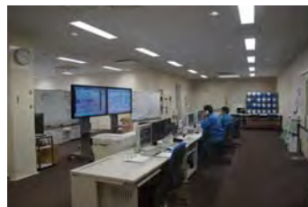
Kawai Water Treatment Plant by PFI Scheme, Yokohama City
