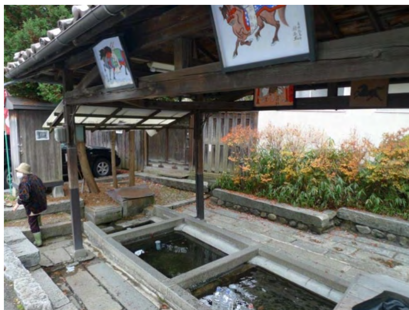
Photo 11. This spring water is currently used in Morioka City. Traditional water grids which are separated for drinking, washing and other purposes from the upstream (November 23, 2010).
