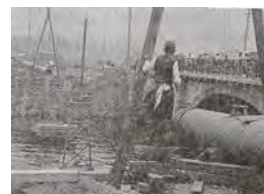
Repair work by utilities (partly subsidized by national fund)
