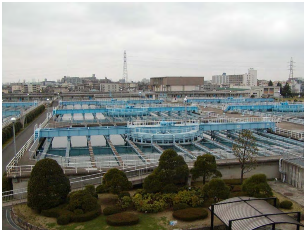
Photo 2. Kanamachi Water Treatment Plant, Bureau of Waterworks, Tokyo Metropolitan Government. It is equipped with advanced water treatment facilities which include rapid sand filtration, high-speed coagulation, flocculation and sedimentation reservoir. It also has power generation facilities, constructed using private financing (April 4, 2004).
