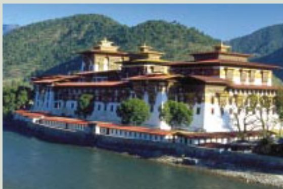
The Punakha Dzong that JOCVs helped restore. To preserve traditional features, their restoration and rebuilding activities included producing a record of the project and giving guidance on building methods that leave the original structure intact. (Photo by Kazuyoshi Nomachi)
