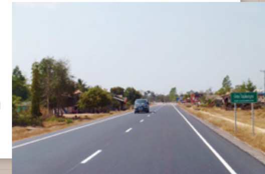
National Route 9, a part of the Mekong East-West Economic Corridor, has been refurbished and improved through the support of JICA.
