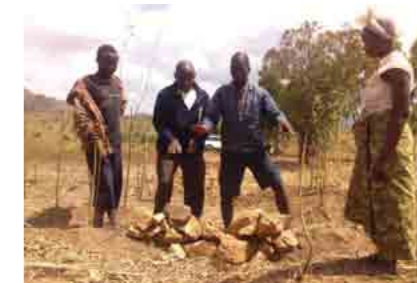
Farmers in Malawi gathered rocks to make a check dam in order to reduce soil erosion from cultivated land on a steep slope. The effect of each small handmade check dam is limited, but it can be increased by having residents cooperate to build a large number of them.
