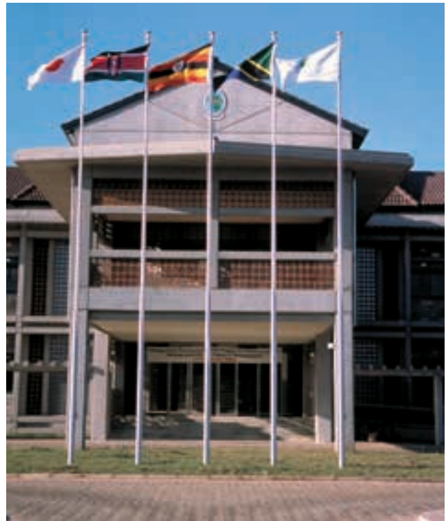
Headquarters of the African Institute for Capacity Development (AICAD) Project
