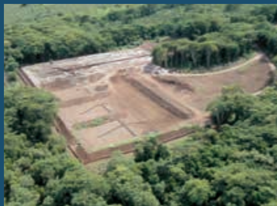
The Tafaigata waste disposal site in Samoa
