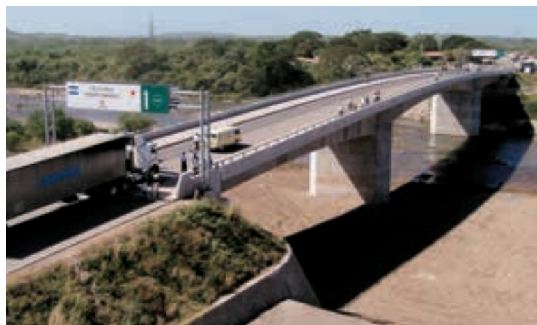
A bridge constructed through the Guasale Bridge Reconstruction Project between Honduras and Nicaragua
