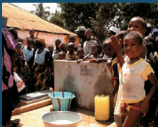
Public water taps constructed at Kalaboui village
