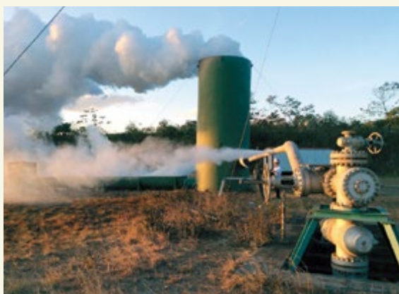
Geothermal well testing
