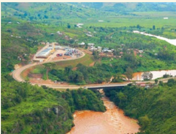
Rusumo International Bridge and OSBP facilities on the Tanzania-Rwanda border
