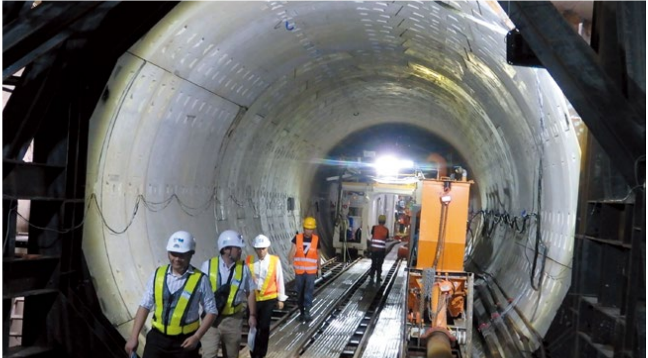
Viet Nam: A construction site of the Ho Chi Minh City Urban Railway Line 1, between Opera House and Ba Son stations. An underground tunnel is being constructed with the shield tunneling method.
