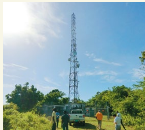
A pylon on which a digital radio antenna will be mounted. A total of 24 such pylons will be constructed throughout the country.
