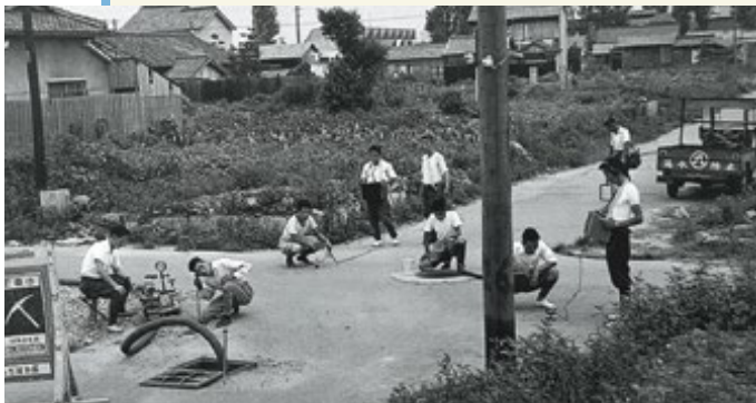
A water leakage check by Nagoya City Waterworks and Sewerage Bureau in the aftermath of World War II, circa 1949.
