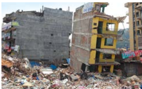
Nepal: Collapsed buildings in the April 2015 earthquake
