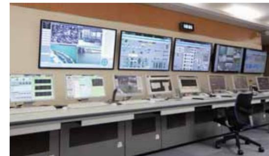
The monitoring and control system integrates and monitors several water treatment plants. Based on know-how which we cultivated during commissioned O&M services, this system has been completely renewed without affecting plant operation.
