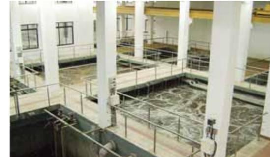
The MBR system ensures space saving. Automatic control and centralized monitoring for water and sewage treatment processes are carried out through PLC and SCADA. The BNR process is applied for denitrification and dephosphorization.
