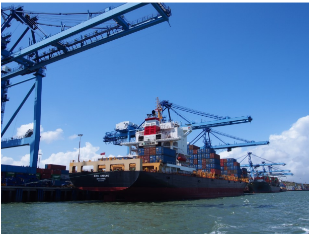
Mombasa Port Development Project-phase (2) in Kenya Photo: JICA
