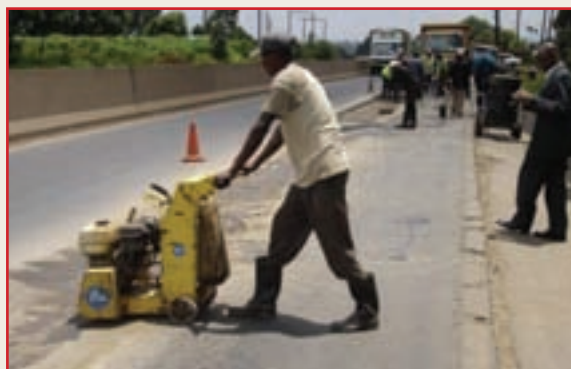
Repair works on Waiyaki way under the SRMMU project.
