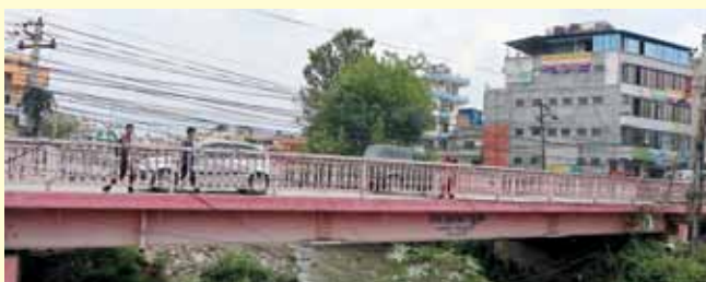
Dhobi River Bridge, Anamnagar, Kathmandu
