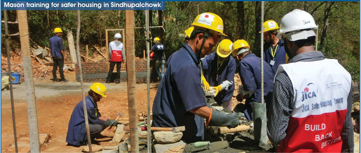
Mason training for safer housing in Sindhupalchowk
