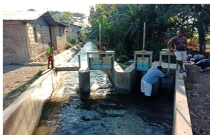
Canal monitoring in Maliana
