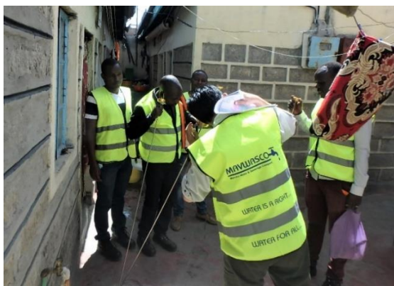
Leak detection on service pipes with listening sticks
