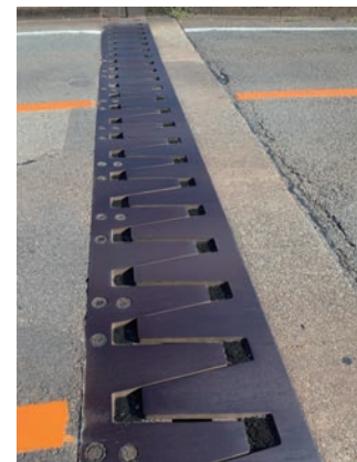
Metal parts allow the bridge to change length.
