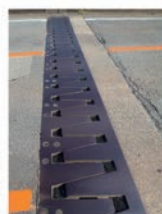
Metal parts allow the bridge to change length.
