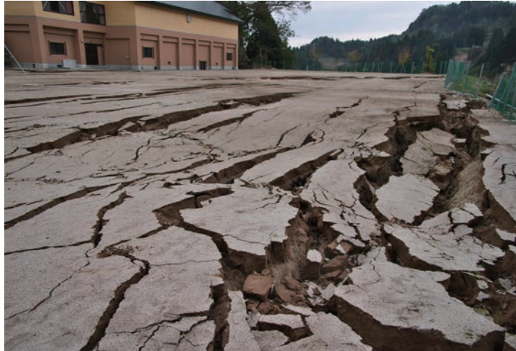
Earthquakes cause cracks on the ground.
