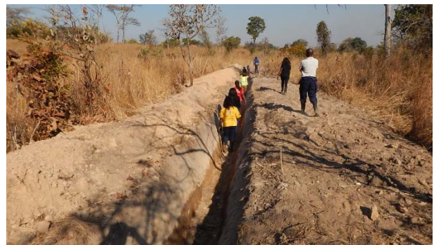
The depth of canal which farmers dug so far is very deep because Farmers tend to choose routes of canal that allows irrigation water to reach the beneficiary area from weir point as quickly as possible without considering heavy labor forth required. Mutundu North, Mutundu Camp, Mufulila District, Copperbelt Province
