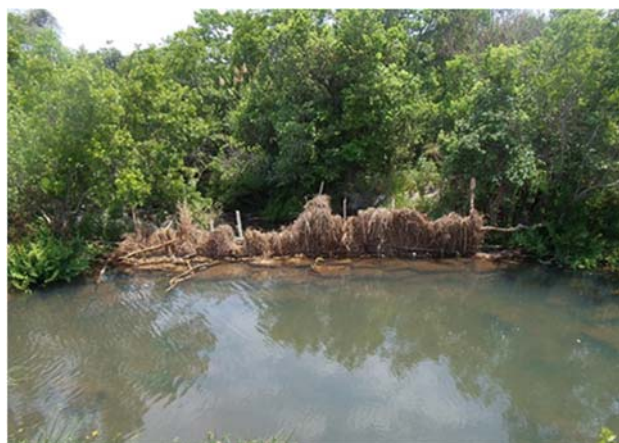
Typical simple weir constructed in large river (Mkushi district in Central Province)
