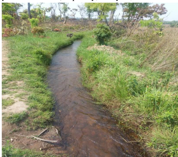
Nseluka Irrigation Site in Mungwi District, Northern Province constructed by COBSI-study. The picture shows main furrow at upper part of the site. Farmers monthly conduct O&M of furrow and the condition is good. Volume of the water is high in the furrow.
