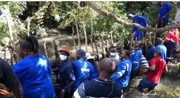
Participants learnt how to construct a simple weir, a entry point of small-scale irrigation development in the field.
